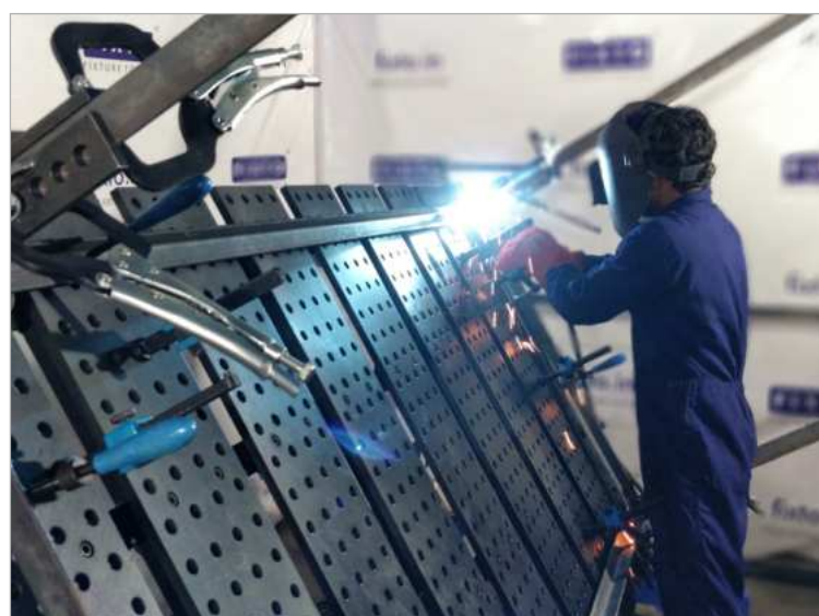
Welding in taper position
